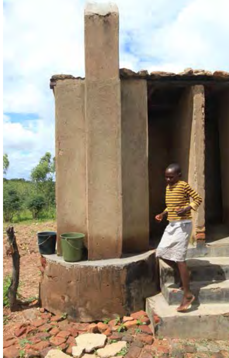
Improved latrines and washing facilities are constructed by Community Health Clubs
