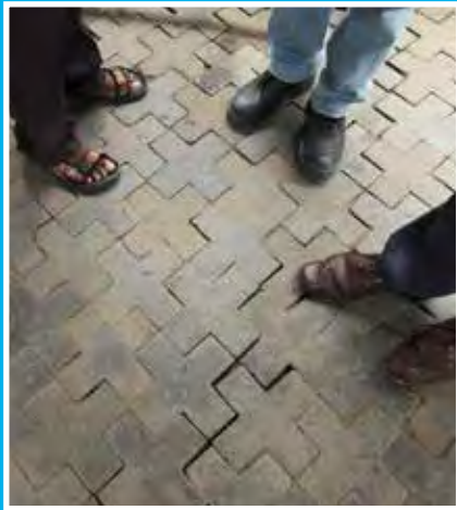
Floor tiles made from sand mixed with melted plastic: a waste management innovation from the Karoi town council
